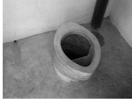
Figure 3b: EcoSan Latrine installed with seating pan
