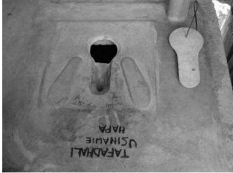
Figure 3a: EcoSan Latrine installed with squatting pan (Photos by EEPCO 2002)
