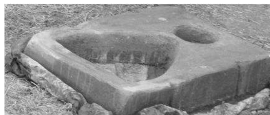
EcoSan squatting pan – Promoted by Water and Environmental Project Management organization (WEPKO). Photo by EEPKO 2007.
