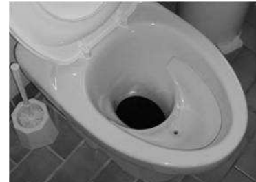
Urine diversion and dry composting of fecal matter atTingvall conference center Sweden. Source Prof Dr. Petter D. Jenssen
