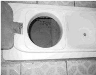
Composting toilet with urine separation (China) – Source: Christine Werner, Patrick Bracken, Florian Klingel
