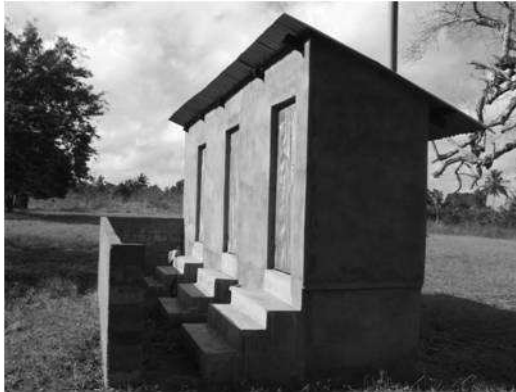
Figure 3: EcoSan School Toilet at Titu Primary school – Kisarawe District Coast region (photo by EEPKO 20006)
