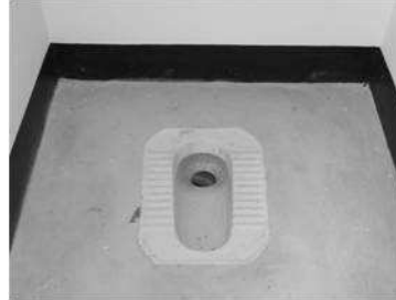
Figure 5: Squatting WC usually used in Tanzania (mostly imported from India and China). Photo by EEPKO 2006 Approximate costs of the WC/pan: Chinese = US $ 6.7, Indian = US $ 7.5
