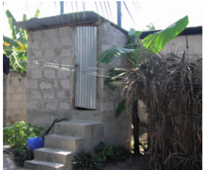
Top: Photo 1: Ecological toilet with urine tank in front and "uwani"
